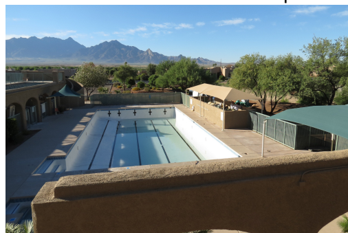
New canopy to cover pumps
