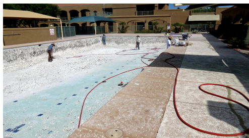
Drilling out plaster base
